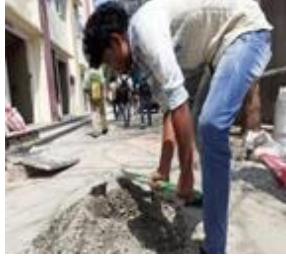
Figure :2- Mixing of concrete
